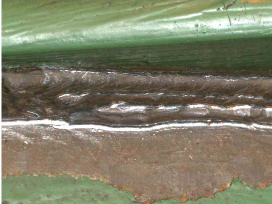
Fig 7 Ultrasonic Peening Treatment of multi-pass weld toe
