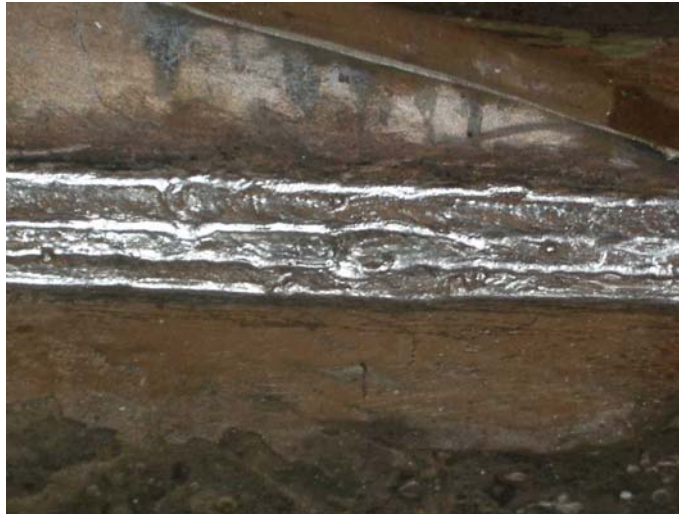
Fig 9 Treatment of weld spatter, multi-pass weld toe and start/stop locations.
